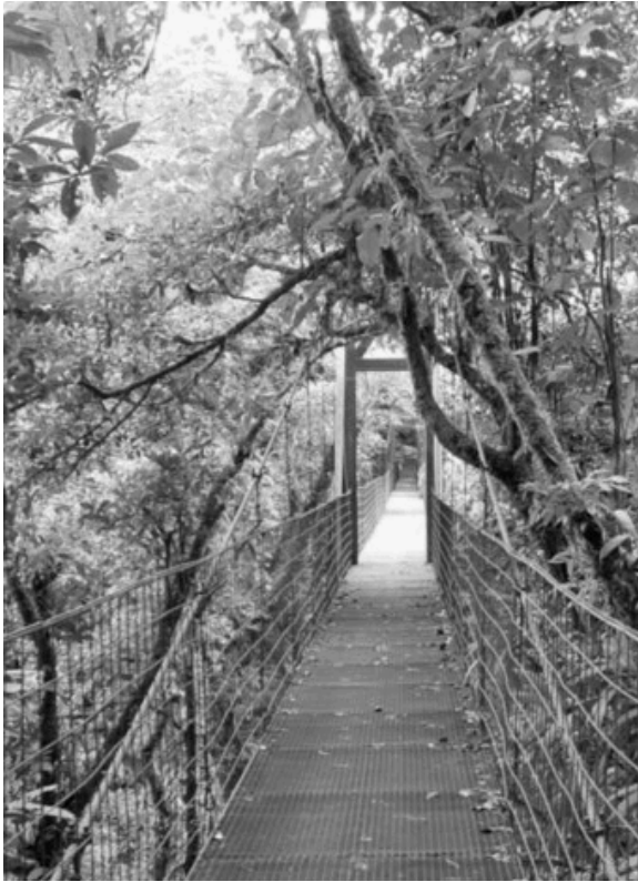
SUSPENSION BRIDGE IN MONTEVERDE, PUNTARENAS, COSTA RICA
